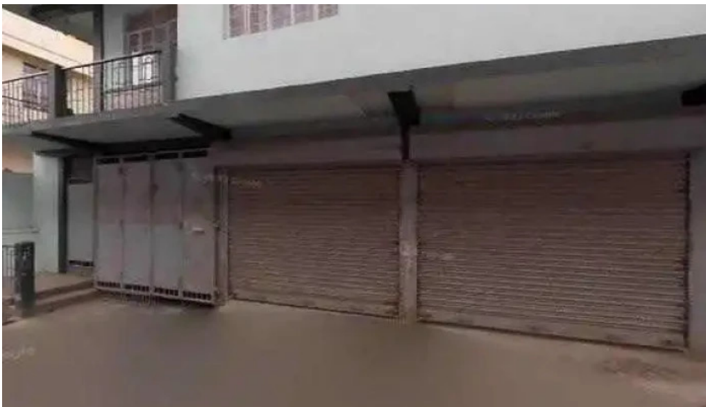
Megsol it solutions company street view 360deg
