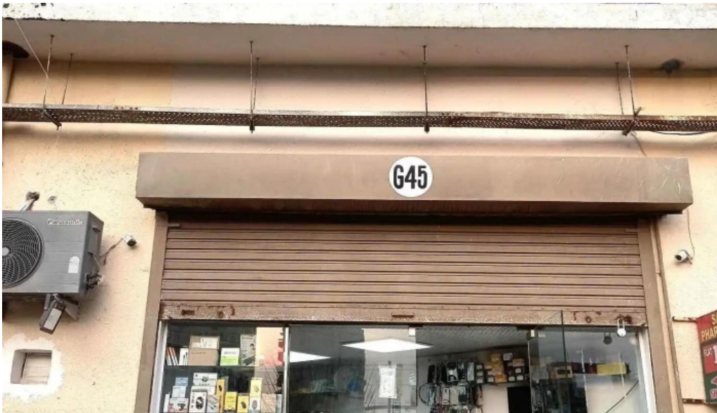
Tech hub 37c exterior
