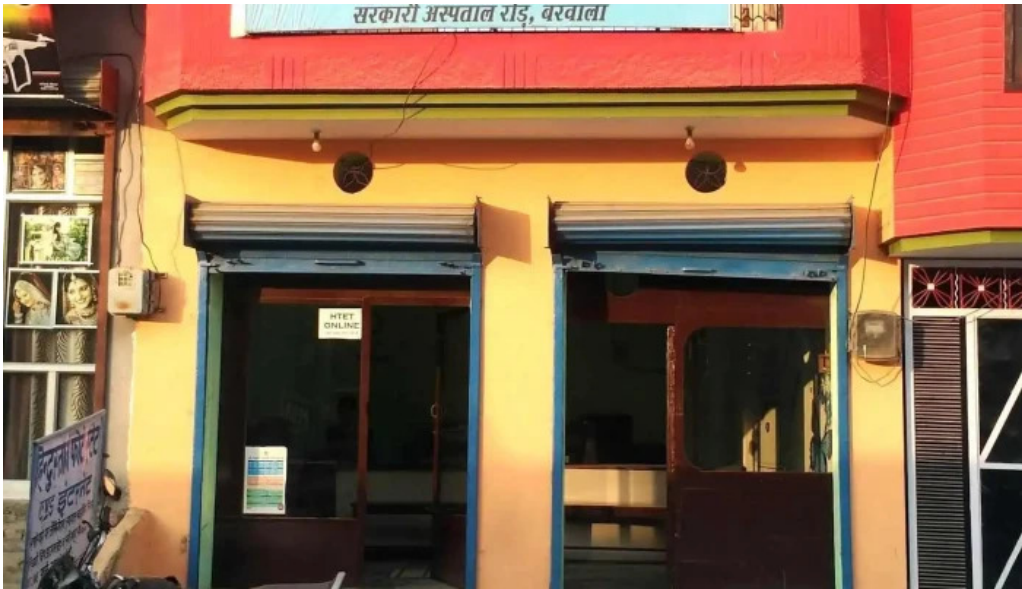
Hindustan photostat csc library exterior
