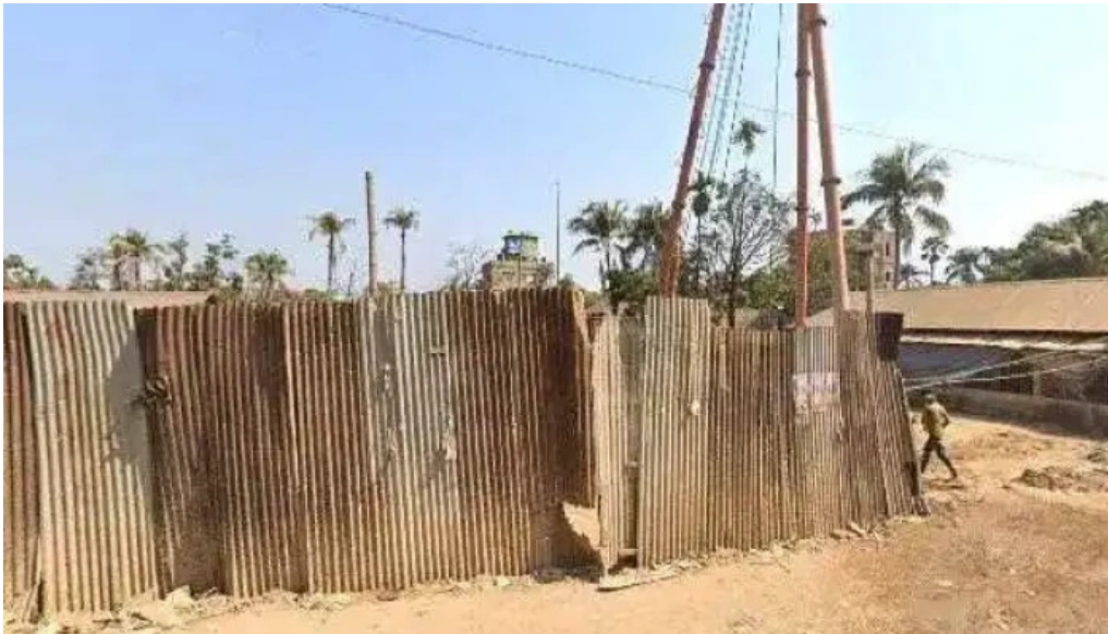
Bappy telecom and computer centre street view 360deg
